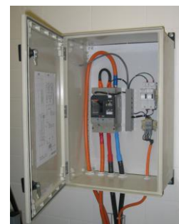
Figure 7: Coffret de protection des batteries
